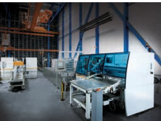
KASTO saws at a buffer station.
