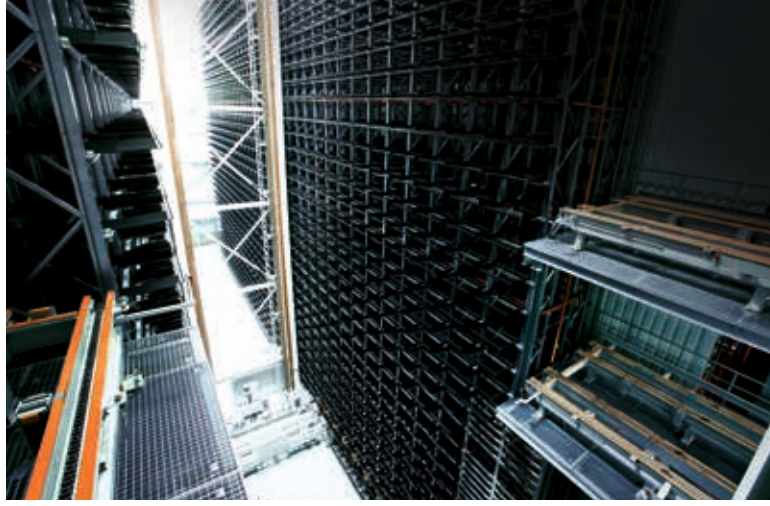
Station over several floors.
