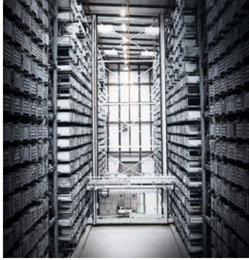
UNICOMPACT in an aluminum extrusion facility.
