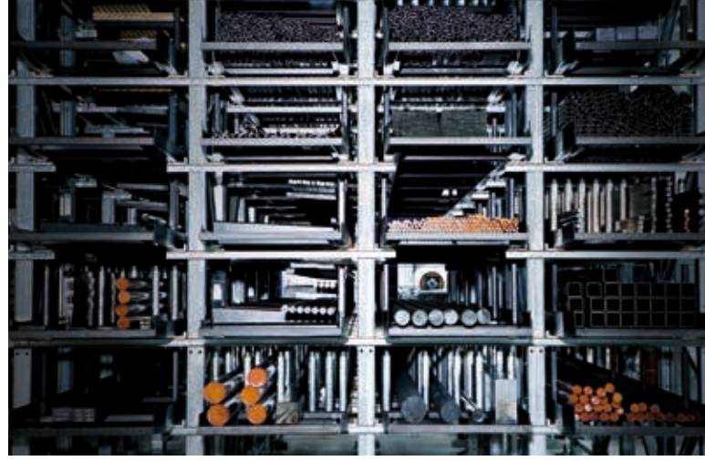
View of the Honeycomb steel structure with cassettes for mixed operation (automatic and standard cassettes).
